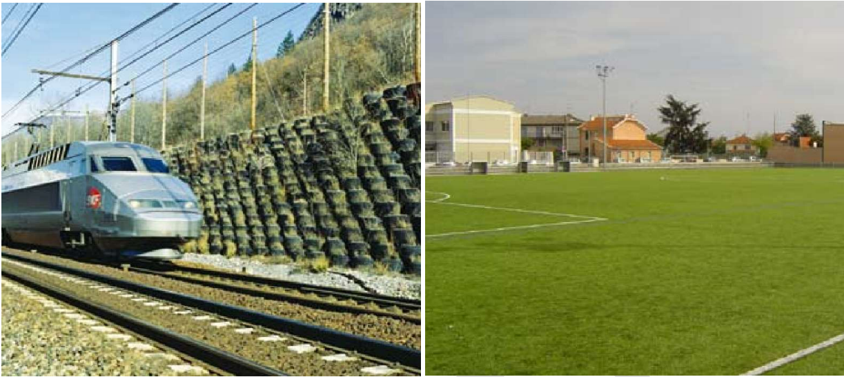
Figure 6. Source: Anti-scrree wall in the Hautes Alpes, France (Aliapur, DR). Artificial turf on playing field, France (Michelin).
